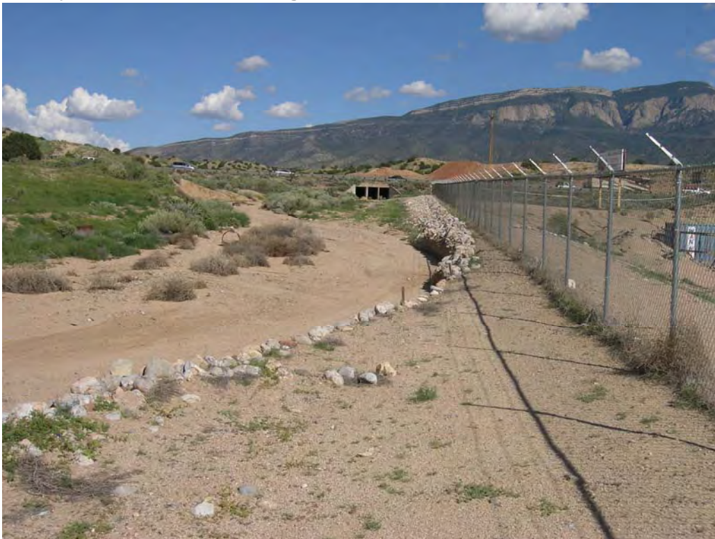
Arroyo meander encroaching on commercial site
