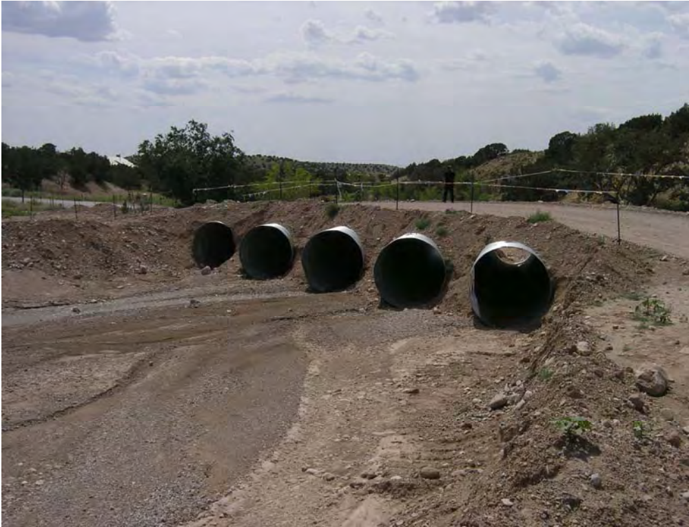
Replacement culverts due to 2006 road washout on Camino de las Huertas
