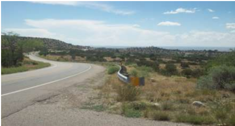
NM 165 Looking West Near the County Fire Station
