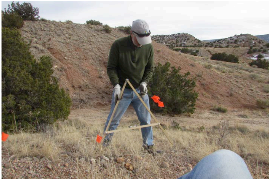
d. Volunteer using an A-frame with small level to mark contours for berms.
