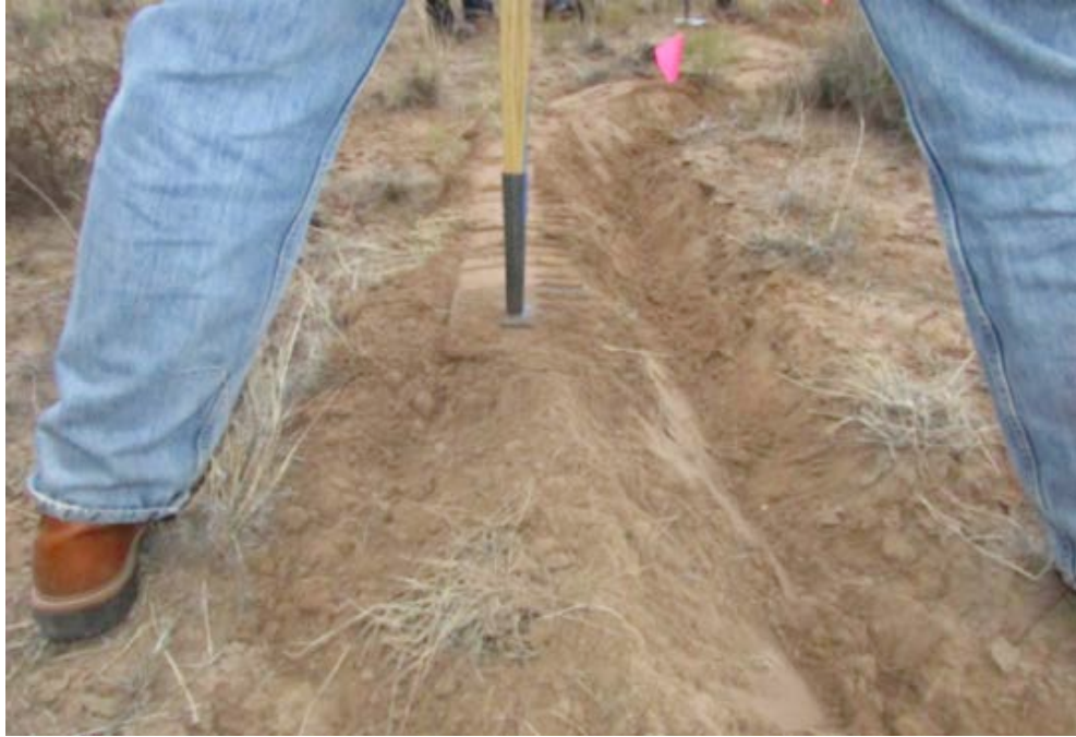
c. Swale and berm being created, using a McLeod Tool.
